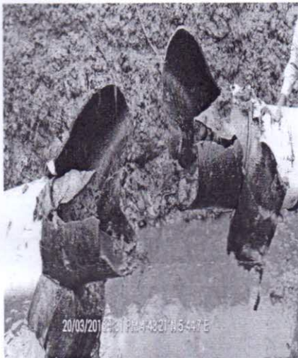
Fig A: picture taken after excavation.
