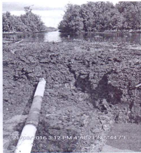
Fig B: picture taken after sectional replacement.
